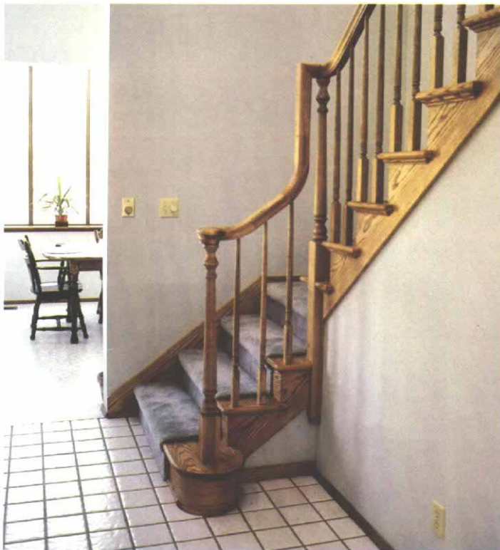
When laying out a balustrade, measuring the components in place works best. Clamp the handrail and fittings in place right on top of the treads to determine where and at what angle to cut them. The finished installation shows a starting newel with a turnout and a two-riser gooseneck that had to be extended because of the location of the landing newel.
