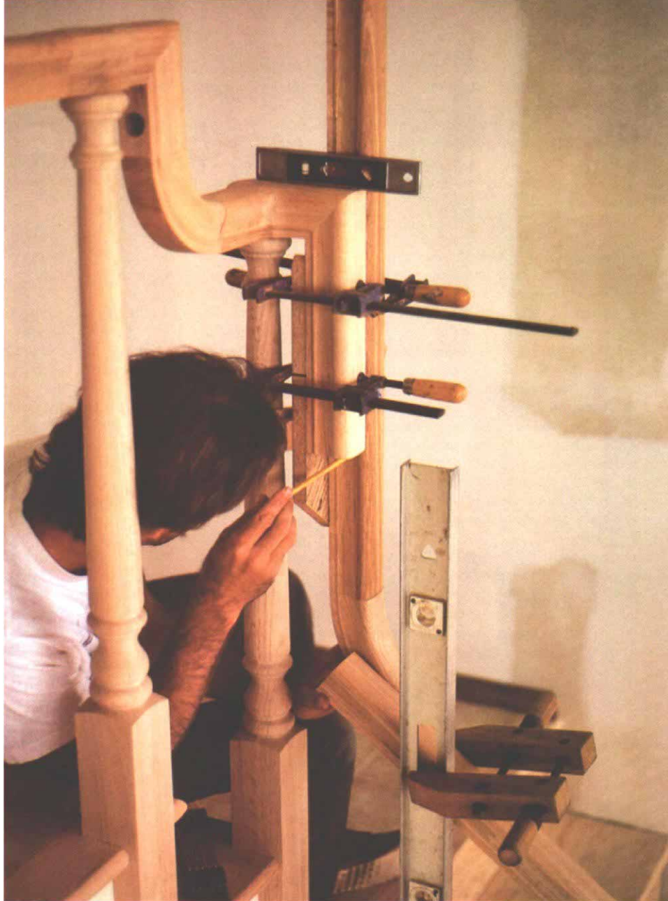
Ready for final assembly, the joining faces are coated with glue, the rail bolt inserted into the adjacent fitting (top left), and the nut and washer started, then tightened, through the large hole on the bottom of the fitting (middle left). Because they make for a smoother assembly, the author prefers hex nuts and a box wrench to the star-shaped nuts supplied with the rail bolts. The match between straight handrail and fittings is never perfect—some fairing is always needed. At left, a 2-in. dia. sanding disc attached to an electric drill is used to smooth the joint. In the photo above, the newel posts have been installed temporarily in order to calculate the cuts for attaching the easing between the gooseneck and straight rail. A section of straight rail has been attached to the easing and lined up with the vertical leg of the gooseneck to help position the easing correctly.
