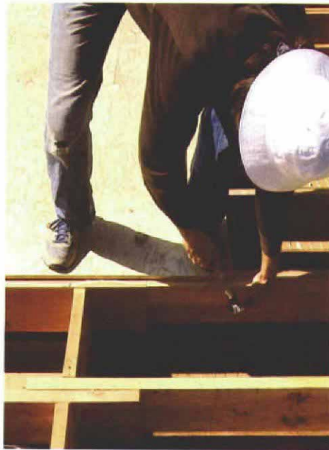
When joists are lapped, you have to add a block to pick up the unsupported edge of a piece of subfloor. There's a V-shaped mark on the plywood to the right of the hammer. It tells the person nailing where the centerline of the joist lies, and the direction it runs.
