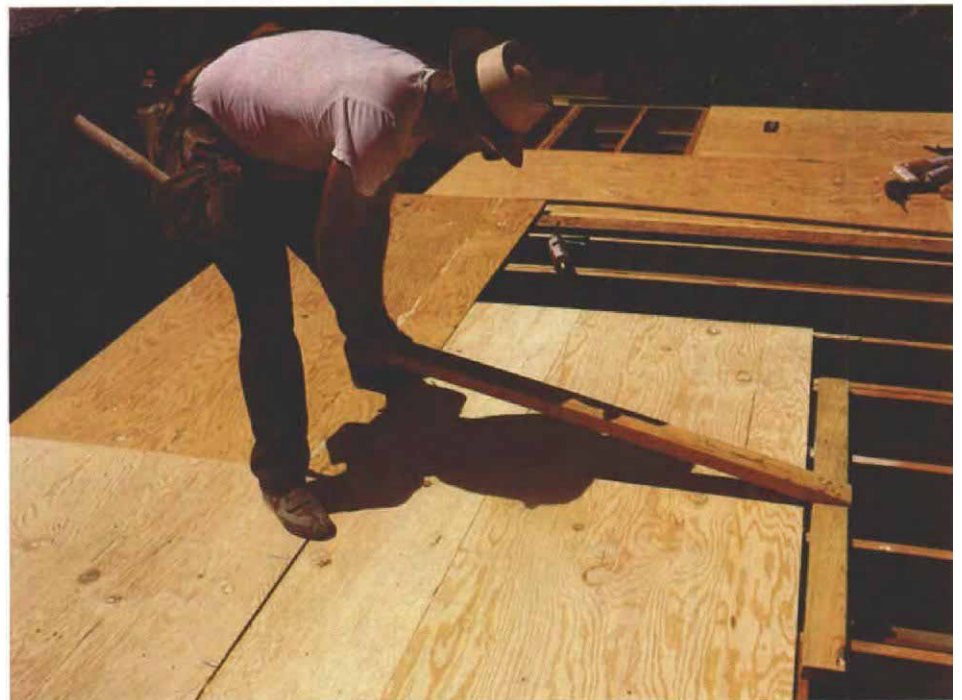
The bump-stick is a T-shaped tool made of framing lumber that can help when you're installing T&G plywood. Align the tongue on the workpiece with the grooves in the installed sheets by standing on them. Then pull on the bump-stick to drive the sheets together.
