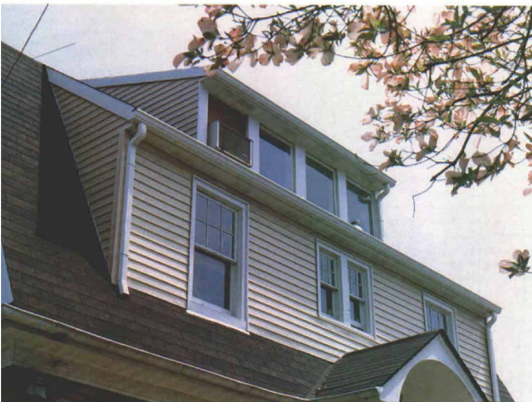
Piggyback shed dormers. Shed dormers are often part of the original design on houses that have a gambrel roof. Here a second dormer was added on top of the first, probably to let more light into the room. For more examples of atypical shed dormers, see pp. 80-81.
