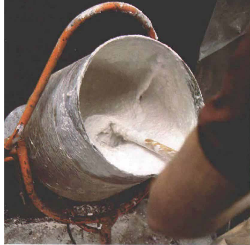
Mixing plaster is a messy business , and adjacent structures or plants have to be protected with plastic sheeting. Once the plaster reaches the consistency of cake frosting, as shown above, it should be mixed for another fifteen minutes before it's applied to the wall.
