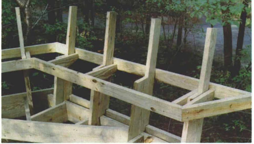
Bench supports built from 2x8s can be trimmed to a width of about 3\frac{1}{2} in. where they form the backrest. The supports should be securely nailed or bolted to the decks supporting structure.
