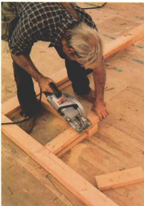
Plating. Peake cuts in the top and bottom plate of a small raceway (left), and tacks each of the two sets of plates together with 8d nails (right) so they can be detailed. One of the first decisions in plating is which walls will run by, and which will butt. Here the long interior wall is a by-wall, and the parallel wall of the raceway is plated the same way.
