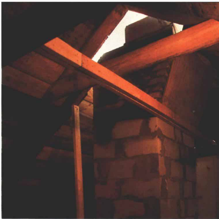
Just below the roofline, the chimney wall shown above changes from 4-in. thick concrete block to brick. Block is much faster to lay up than brick, but it's usually used where appearance isn't important. The brick wall has been corbeled out against a temporary plywood form, enlarging the chimney above the roof and also centering it on the ridge. From this stage on, a good working platform on the roof is essential, right.
