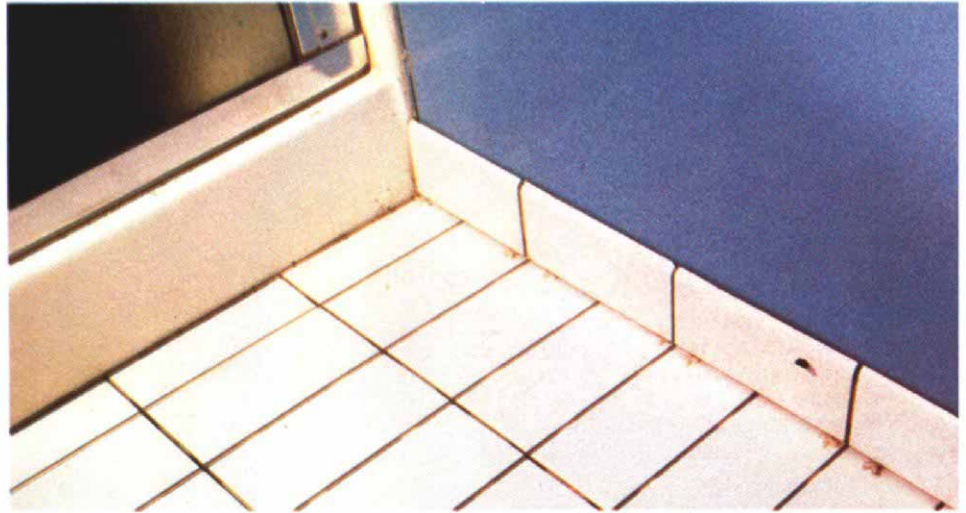
Trim tiles. It's easier to apply the epoxy to individual trim tiles, left, than it is to comb the mastic onto the wall. Trim tiles are temporarily held in place by plastic spacers, below, while the mastic sets up. Notice that the trim tile on the left has been shortened to match the width of the field tiles adjacent to the shower enclosure, so that the grout lines on floor and trim align.
