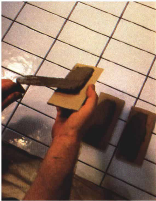
Trim tiles. It's easier to apply the epoxy to individual trim tiles, left, than it is to comb the mastic onto the wall. Trim tiles are temporarily held in place by plastic spacers, below, while the mastic sets up. Notice that the trim tile on the left has been shortened to match the width of the field tiles adjacent to the shower enclosure, so that the grout lines on floor and trim align.
