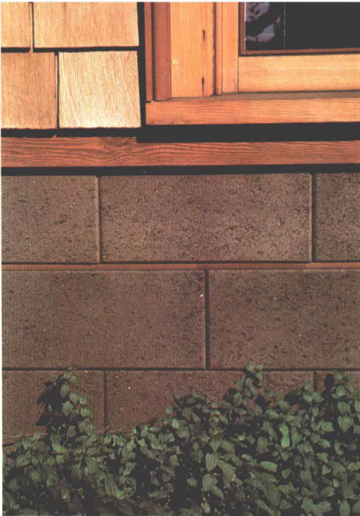
A quarry-tile inlay makes a thin red stripe around the house. The blocks have been sandblasted and sealed, revealing their volcanic aggregate.
