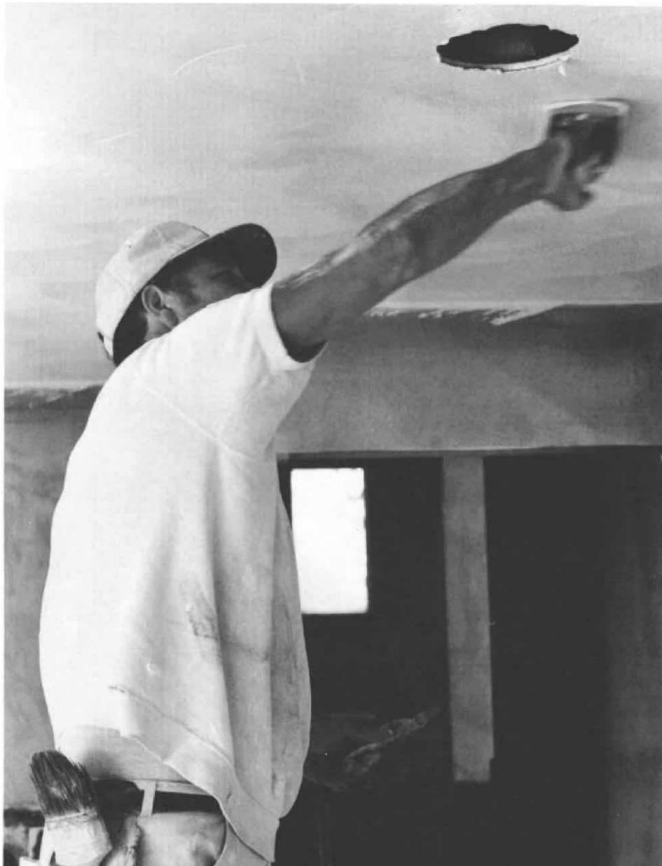
Applying the plaster. Above, the last of a batch of finish coat is about to be hawked and applied to the scratch-coated wall in the background. Learning how to handle the fluid mix takes practice. Speed is essential, since the plaster sets in less than an hour. Once applied, each coat is either floated smooth or textured. Using an overlapping circular motion, below, and keeping the float clean and wet help speed the work. Lighting fixtures and trim are installed after the finish dries.
