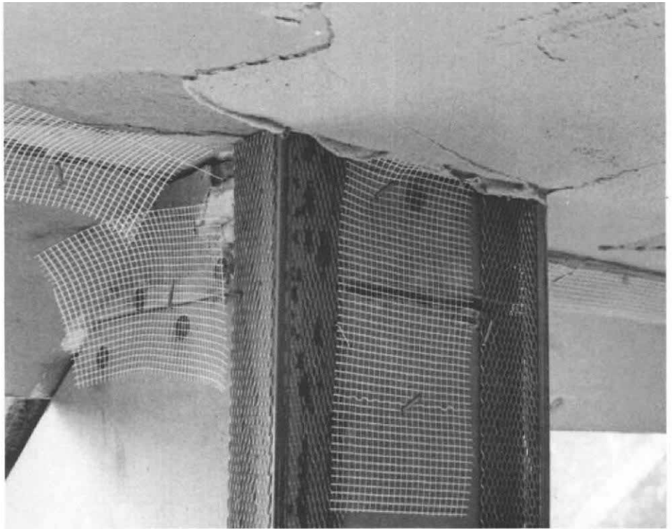
Preparing the surface. Before the first coat of mud goes on, corners, above, are beaded with metal or plastic grounds. All joints are reinforced with fiberglass mesh-tape. The plaster compound can be mixed using either a commercial rig, below, or a powerful electric drill and spade. Water must be clean enough to drink, and solid should always be added to liquid.
