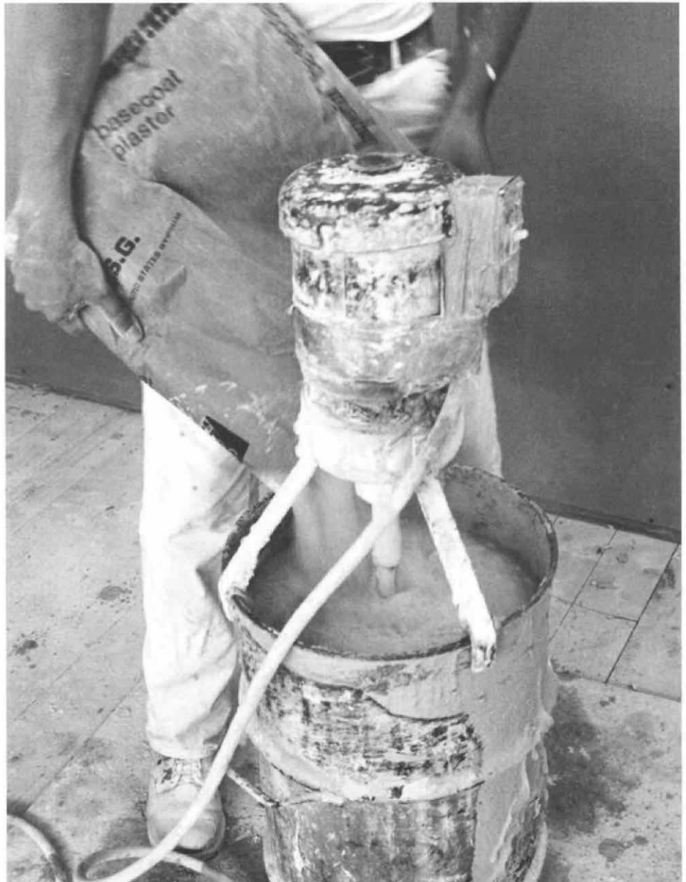
Preparing the surface. Before the first coat of mud goes on, corners, above, are beaded with metal or plastic grounds. All joints are reinforced with fiberglass mesh-tape. The plaster compound can be mixed using either a commercial rig, below, or a powerful electric drill and spade. Water must be clean enough to drink, and solid should always be added to liquid.
