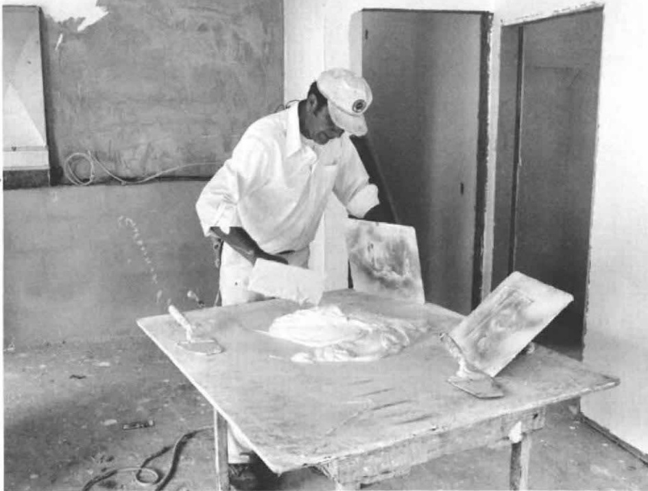
Applying the plaster. Above, the last of a batch of finish coat is about to be hawked and applied to the scratch-coated wall in the background. Learning how to handle the fluid mix takes practice. Speed is essential, since the plaster sets in less than an hour. Once applied, each coat is either floated smooth or textured. Using an overlapping circular motion, below, and keeping the float clean and wet help speed the work. Lighting fixtures and trim are installed after the finish dries.
