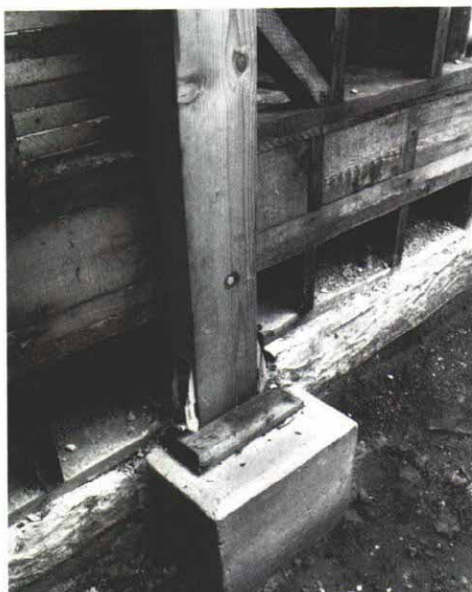
An independent post-and-beam skeleton. Lag-bolted to the first-floor framing, 4x8 posts rest on individual piers (drawing and photo, left). Atop the posts, 4x16 beams form a structural perimeter to hold floor joists and walls of the second story (inset, above). The badly deteriorated original stucco finish has been removed from the first-floor walls (top). They will be restuccoed. The exterior on the new second story will be board and batten.
