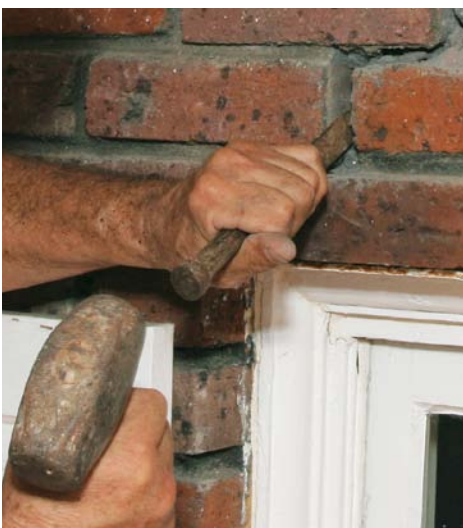
Clean the drilled joints with a cold chisel. Don't chisel straight in or you'll risk loosening the bricks. Rather than pounding the chisel, just tap it and take out a little mortar at a time to avoid damaging the wall.
