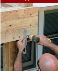
Hangers may need extra support. Whether you're using sloped joist hangers or stringer hangers (shown), dropped staircases usually require additional lumber to provide full fastening for the hardware. Here, the 2x10 rim was furred down by the width of a 2x4 spacer so that all eight fasteners had backing.
