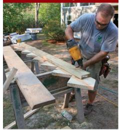
Sister to increase the span. Notched 2x12 stringers have a maximum span of 6 ft. If approved by your inspector, however, this span can be extended by nailing 2x stiffeners to the uncut portion of each stringer.
