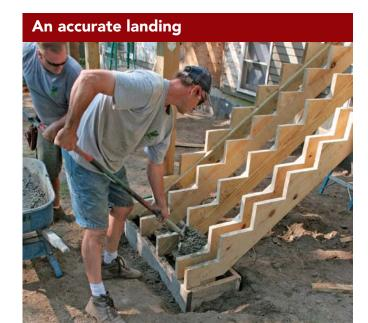
**Pad comes last.** After final plumbing and leveling are complete, shovel concrete into the pad formwork. Once the concrete has cured, strip the form and add wedge anchors through the cleat to anchor the base of the finished stairway.
