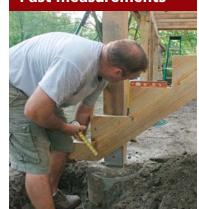
Stringer sets the pad. With the pattern stringer cut, held in position, and leveled, it's easy to measure down to determine the desired height of the concrete formwork that will be installed below.
