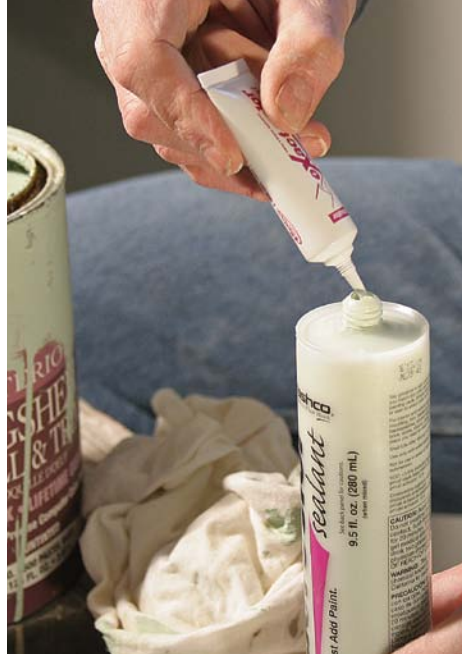
Add activator to the tube and shake. The activator causes the caulk, which is very liquid until now, to thicken.
