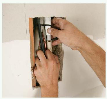
Condensate line runs downhill. Condensation produced during cooling mode is drained to the outside or to an interior drain through a 5/8-in. flexible hose. The hose should slope a minimum of 1/4 in. per ft. for its entire length. When there's no way to drain the water via gravity, a condensate pump within the indoor unit or mounted externally can pump the condensate outside or to a drain.
