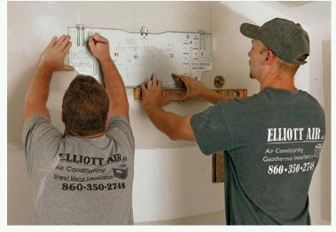
Connections require access. The indoor unit's short lengths of refrigeration tubing and condensate line must be extended to reach the outdoor unit. If the unit is on an outside wall, the extended lines are run on the outside of the building. If the unit is on an interior wall, either the lines need to be roughed in before the drywall is hung, or a hole needs to be cut to extend them.
