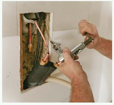
**Reflare the fittings.** The copper refrigeration lines have flare connections. The line sets come preflared and with their own flare nuts, but manufacturers recommend removing these nuts and reflaring to accommodate the flare nuts that come with the indoor and outdoor units.
