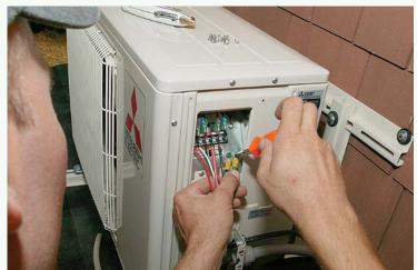
Power requirements are reasonable. Powered by a 20A or 30A circuit, depending on its Btu output, the outdoor unit gets its energy from the disconnect switch through conductors run within a flexible, watertight conduit called a whip.
