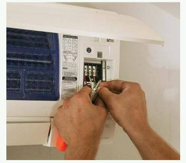
**Power comes from the outdoor unit.** The indoor unit is powered by the outdoor unit through a 14-ga. four-conductor cable. The stranded cable is as flexible as an extension cord, so it's easy to run it and to make the connections. Some versions have reinforced UV-stabilized jackets, so they can be left exposed without a protective conduit.
