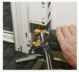
Outdoor connections look like indoor connections. The copper refrigeration lines running from the indoor unit are connected to the outdoor unit with flare fittings. As before, the flare nuts installed on the line set are removed and replaced with the nuts provided by the minisplit manufacturer.
