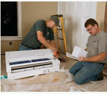
Made for easy mounting. Using the instructions to determine the right location, the installer drills a 3-in. hole for running the refrigeration lines, electrical cable, and condensate tubing to the outside. The bracket is then leveled and mounted the specified distance from the hole. The bracket should be attached to two studs.
