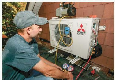
**Evacuating the line set** to prevent problems. Before the service valves are opened and the 410a refrigerant in the outdoor unit is released, the refrigeration lines must be evacuated of air and water vapor with a vacuum pump.
