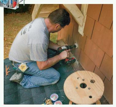
Line sets should take a direct path. Pairs of insulated soft copper tubing make up the refrigeration line set. In this installation, the line set, four-conductor cable, and condensate tubing run from the indoor unit toward the outdoors through an attic crawlspace. The bundle of tubes and wire requires a 3-in. hole that will be sealed later with duct-sealing compound for weathertightness.
