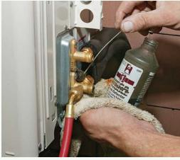
Checking for leaks. After the copper lines are connected, they're pressurized to about 300 psi with nitrogen to test for leaks. A manifold gauge should show steady pressure. The fittings are then coated with a refrigeration-specific soap solution. Any bubbles around the fitting indicate a leak.
