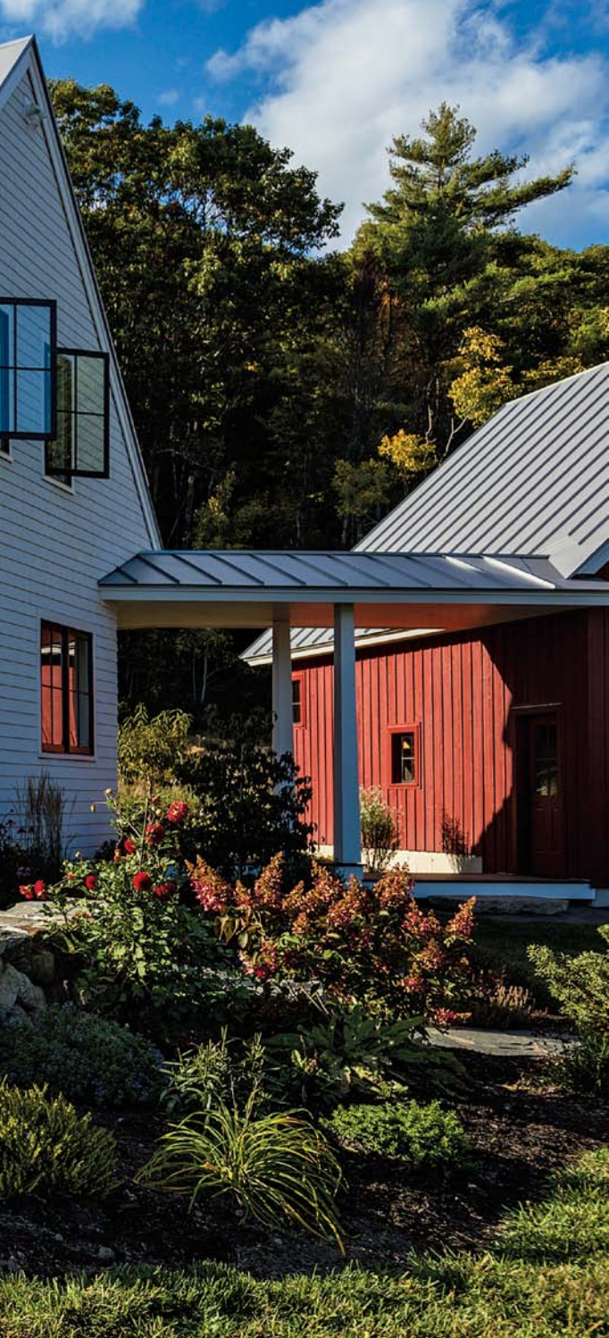
Covered connection. A sheltered walkway links the house's back entrance with the garage, about 20 ft. away. LVLs held up by tapered columns support the roof.
