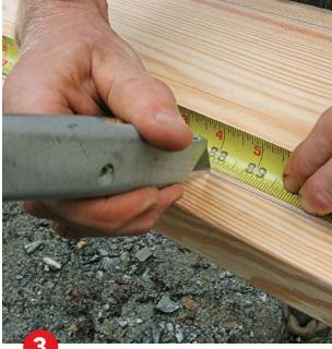
Follow the line. Measure from the intersection of the chalkline and plumb cut—starting from the 1-in. mark for accuracy—to mark the rafter length. Adjust this line by half the thickness of the ridge to mark the plumb line that represents the sheathing's outside face.
