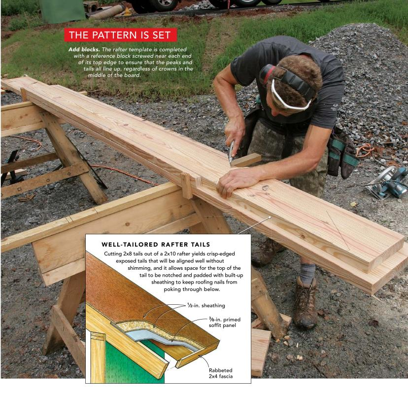
between walls and roof when the layout of the angles is based only on the 6 in. of wood that is directly in contact with the rafter square. Snapping your reference lines eliminates the inaccuracies.
