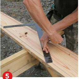
Add the overhang. Reference your framing square off the plumb cut of the bird's mouth to calculate the desired amount of overhang, which is measured perpendicular from the bird's mouth plumb cut.
