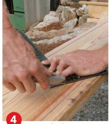
The bird's mouth is 6 in. wide—the combined width of the top plate and the wall sheathing—and referenced off the line that marks the rafter length.
