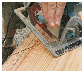
**Start with the bird's mouth.** Penciled-in arrows ensure that the seat and plumb cuts are made on the right side of the knife line. Stop the sawblade where the lines intersect to avoid overcutting.
