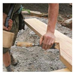
**Finish up with a chisel.** A few whacks on the end of a sharp chisel make quick work of removing the waste from the corner of the bird's mouth.
