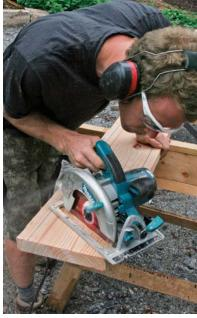
Mark the ridge plumb cut. Align your framing square to the chalkline on the appropriate numbers—the 8-in. and 12-in. marks for this 8-in-12 pitched roof—and scribe a line for the ridge plumb cut. I use a utility knife for all cross-grain marking because the knife line is more accurate than the sharpest pencil line, and it shears off cleaner when cut with a circular saw.
