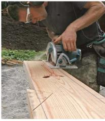
**Next come the cutouts.** Working from the plumb cut in, cut along the pencil lines to create the clean-cut 2x8 rafter tail.
