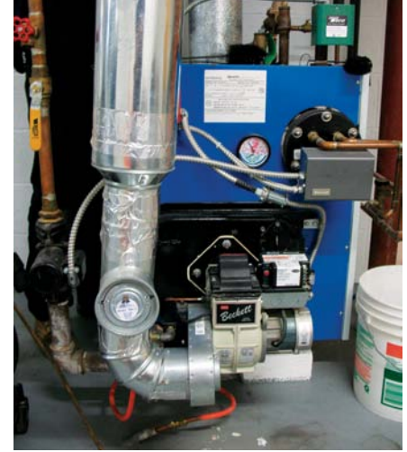
Dedicated combustion air. In tight houses, boilers and similar appliances should be supplied with air through a duct leading directly to the outside.
