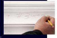
suring each room is important, as it ensures that you don't miss any sections. Use this cutlist to rough-cut the trim. If some of the boards have knots in the middle, use them for the shorter pieces. This ensures that the best long boards remain intact for the longest runs.
