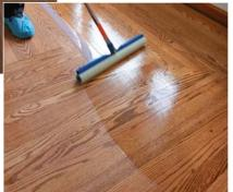
of stain, we combine them in one bucket to ensure that the color is uniform. We apply the stain with a lint-free cloth, then wipe the excess before it dries in place.
