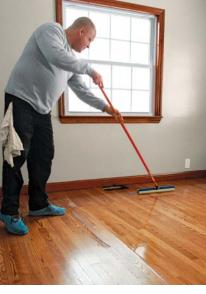
Retouch the curves. Remove the perimeter curve marks by feathering the finish from the edges of the room inward, wringing excess from the T-bar by pressing it firmly on the unfinished part of the floor.
