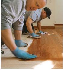
A two-person staining team. Working on padded hands and knees to prevent moisture spots that will keep the stain from penetrating evenly, the first person wipes the stain on using a folded cotton cloth while the second person follows behind, using another cloth to work the stain into the wood in a firm, circular rubbing motion.
