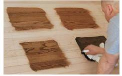
Use the floor as the sample board. The most accurate way to decide between stain colors is to apply the stain options right to the floor after the first or second pass with the belt sander. They can then be sanded out with the next pass.
