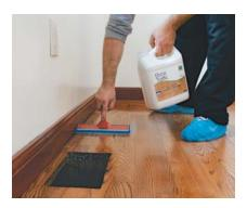
Edges come first. Working just ahead of the person applying finish with the T-bar, coat the perimeter of the room by pouring a thin line of finish directly onto the floor, then spreading it with a handheld applicator pad.
