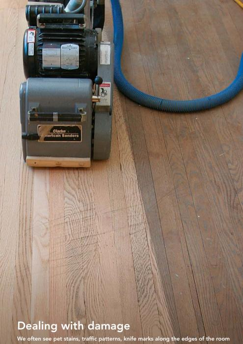
left from the carpet installation, and missing wood or abandoned registers. Our first choice is always to sand out the damage if we can, but damage often extends beyond the missing, scratched, or dented wood.
