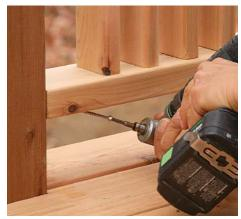
Fasten the bottom. After removing the blocks spacing the rail off the deck surface, drive the lower screws. The clearance is tight, but a right-angle drill attachment helps to set them.
