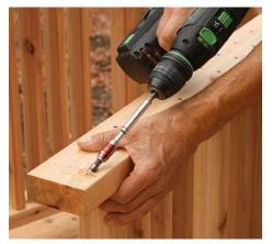
Drill the rails for toe-screws. The rails are screwed to the 4x4 posts from the bottom to hide the 2½-in. stainless-steel screws. Drill the holes at about a 60° angle through the bottom ends of the rails.
