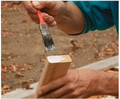
Cutting 70 balusters calls for precision. A stop block on a miter saw helps to make repeated cuts quickly and accurately. Seal the end grain with Anchorseal (uccoatings.com), a wax-based coating meant for end grain. Brushing it on the baluster ends reduces water wicking and discoloration.
