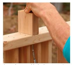
Screw the center blocks. To maintain the 4-in. spacing between the cap rail and the railing section below, fasten 2x4 blocks with 21/2-in. stainless-steel screws. Like the posts, the tops pitch 3° for drainage.
