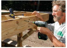
**Tie the joists together with blocks.** Spaced with a scrap of post material, screw two blocks of joist material between the outer pair of joists using 6-in. HeadLoks.
