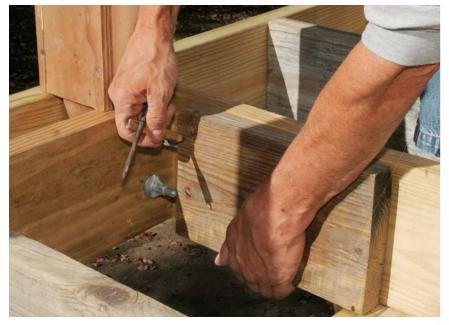
**Install a 16-in. block behind the post.** This block resists outward forces. It's being marked for notches to clear the installed ThruLocks.
