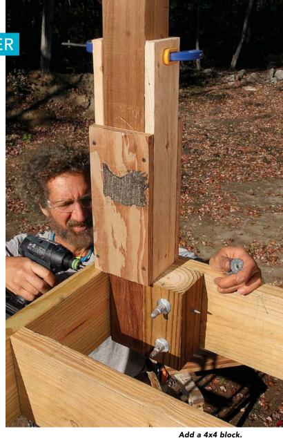
Block the post parallel to the rim. A 2x block fastened on the inside of the rim joist between the post and the next joist using 3-in. decking screws resists sideways loads.
