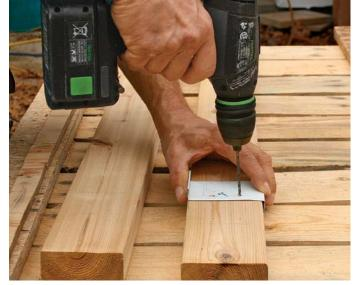
Use a template made from aluminum coil stock to drill the rail sections. The two holes in the template are half the baluster thickness in from the edge. Align the template edge with the baluster-edge marks on the rails to center the holes in the balusters.
