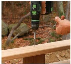
Make the cap rail from straight decking boards. Because the tops of the posts are pitched slightly, the cap rail slopes outward to shed water. Screw the cap rail down with stainless-steel trim-head screws.
