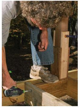
**Tie the joists together.** Using 6-in. HeadLok screws, secure a piece of blocking to give the post lateral stability.
