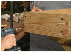
**Secure the rim joist.** Screw the rim joist into the ends of the joists on each side of a post position with 6-in.-long HeadLok screws. The screws need pilot holes before being driven into the ends of the rim joist to prevent splitting.
