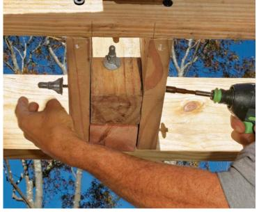
**Tie the assembly together.** A pair of ThruLok bolts locks the 4x4 block between the 2x blocking to reinforce the post.
