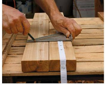
**Transfer the layout.** Pin the elastic to the shorter rail so that the end marks align with the end of the rail. Snap it a couple of times to equalize it, then transfer the baluster position marks.
