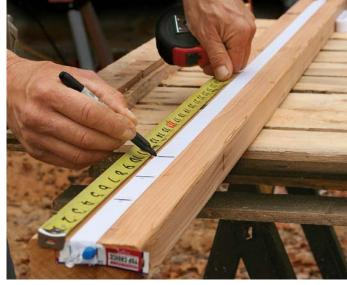
Mark the template. With one end pinned, stretch the elastic about 1 ft. longer than the longest rail. Relax it about 10 in., and pin the other end. Snap it a couple of times to equalize the stretch, then mark the ends of the longest rail and the baluster spacing.
